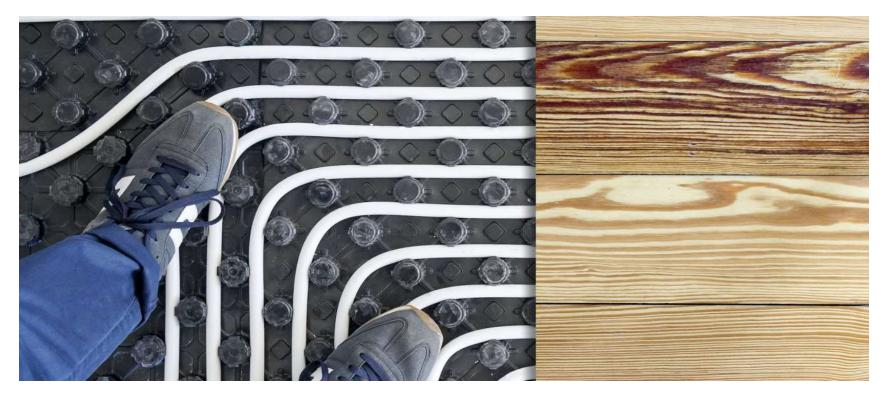
Due to the numerous radiant heat systems, be sure to follow specific manufacturers installation instructions. Regardless of which system is used, overall temperature must not exceed 80 degrees F. Floor temperature should not vary more than 3 degrees F throughout the entire area of the floor.
